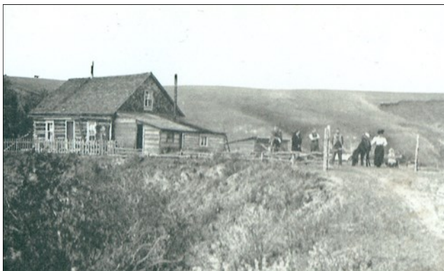
Two-story spruce log house belonging to early rancher-homesteaders, Cutler and Present, along the Three Hills Creek, built from nearby stands of spruce.
